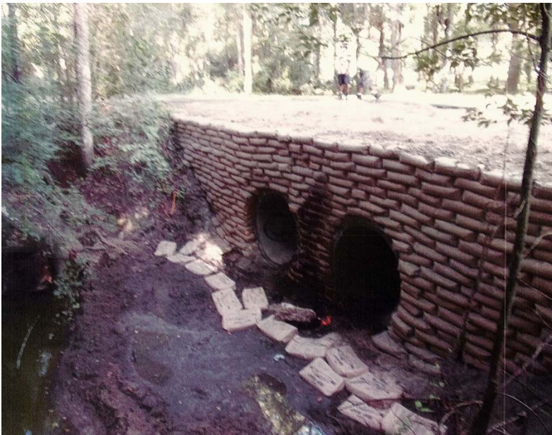
After the Repairs
